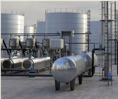
Edifici industriali Industrial buildings
