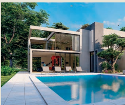
Bordi piscine Poolside
